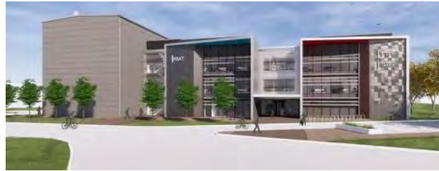
H3AT - tritium research facility
